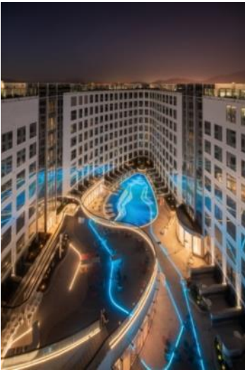
Inner Courtyard with Pool Deck
